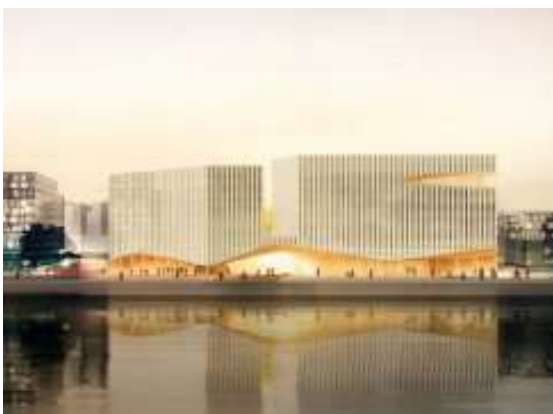
Wood City, Supercell, Helsinki
